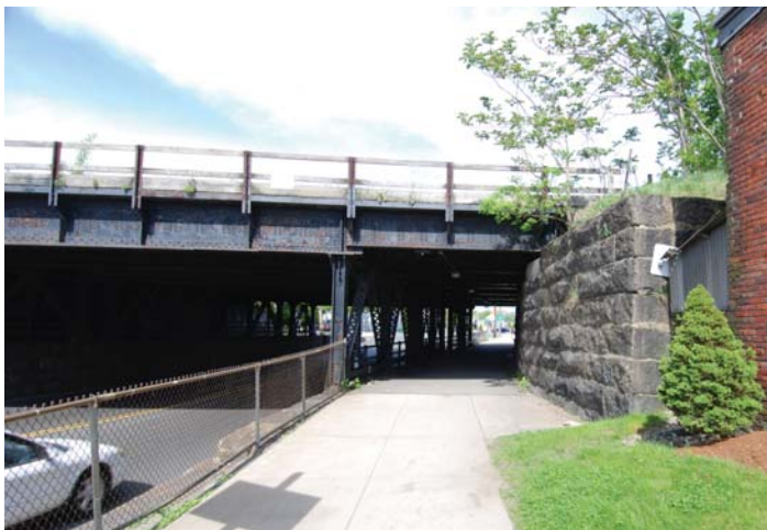
View of existing sidewalk along Washington Street, looking east from Joy Street.
