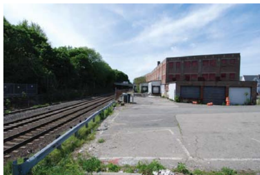
Photo showing the approximate site of the station in the foreground and the city-owned building beyond.
